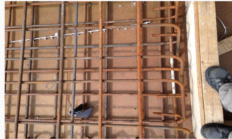
BLL PERIPHERAL TIES AT SLAB FREE EDGE
